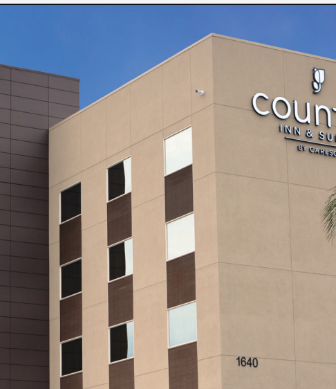
PEBBLE BEACH 1.5 aggregate size to produce a uniform medium sand finish (NOTE: this texture used to be called Pebble Beach Fine)
